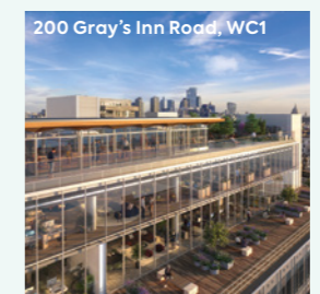
200 Gray's Inn Road, WC1
